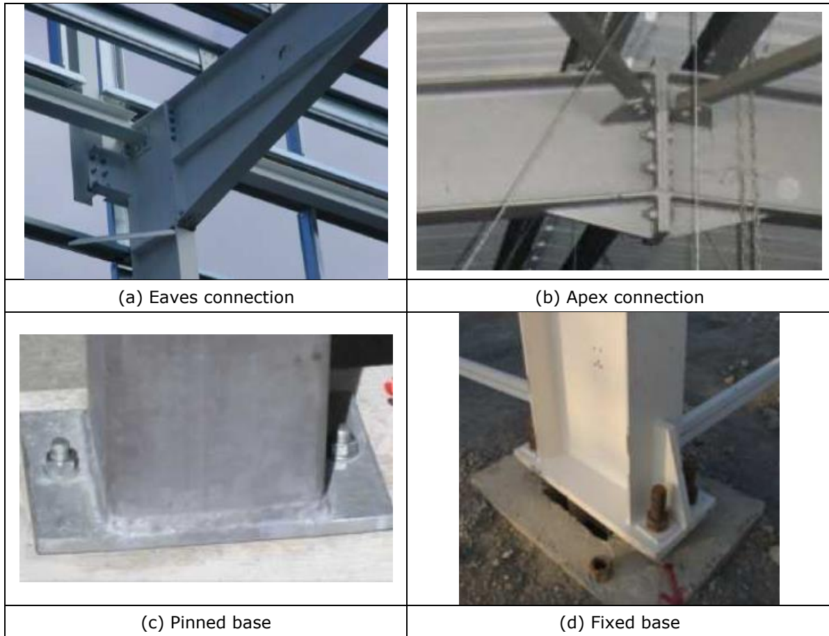
Figure 12: Typical connections in a portal frame (photos)
