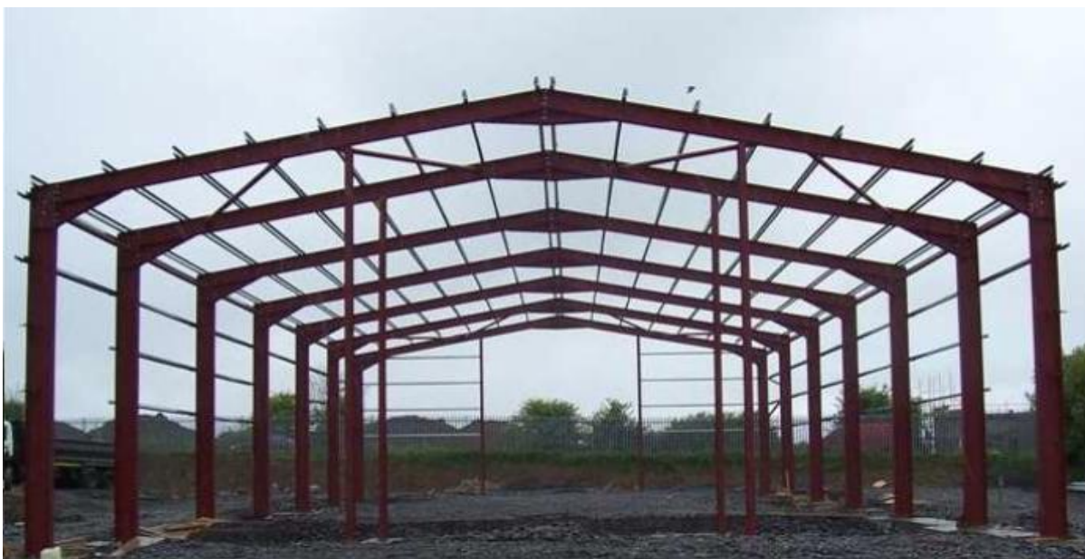
Figure 3: Portal frames with hot rolled sections
