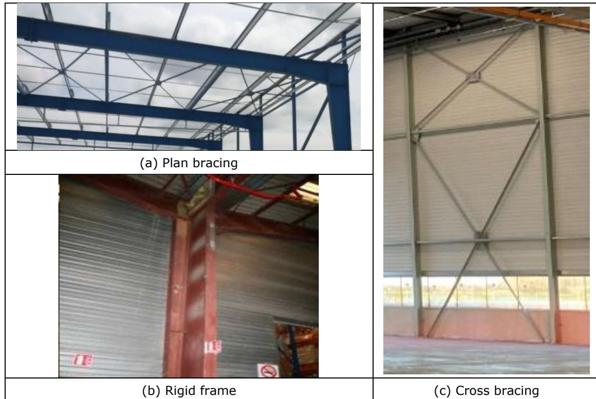
Figure 10: Bracing systems for single-storey buildings
