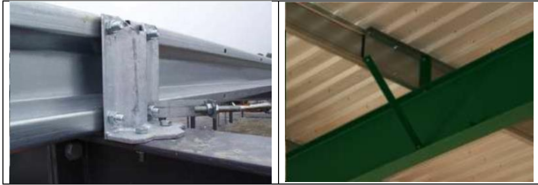
Figure 22: Typical connections for cold-form sections
