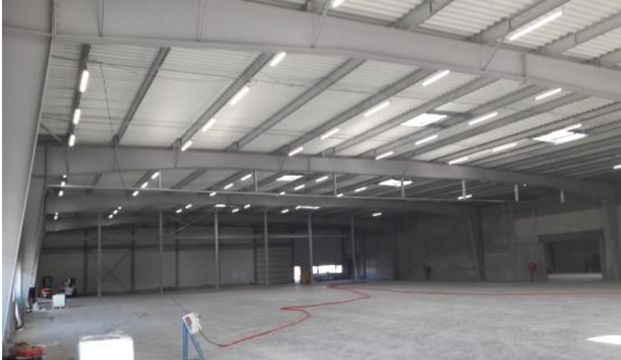
Figure 4: Portal frames with welded sections
