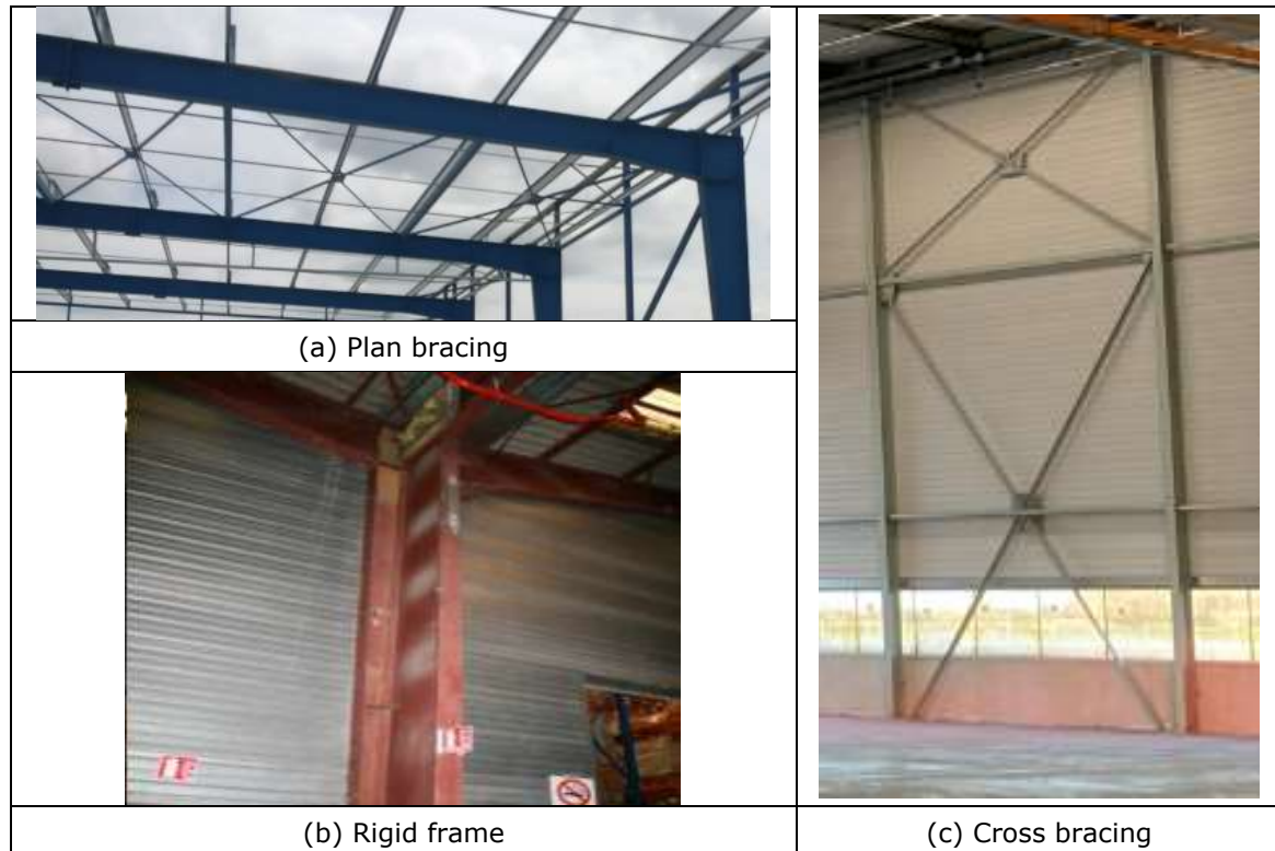
Figure 10: Bracing systems for single-storey buildings
