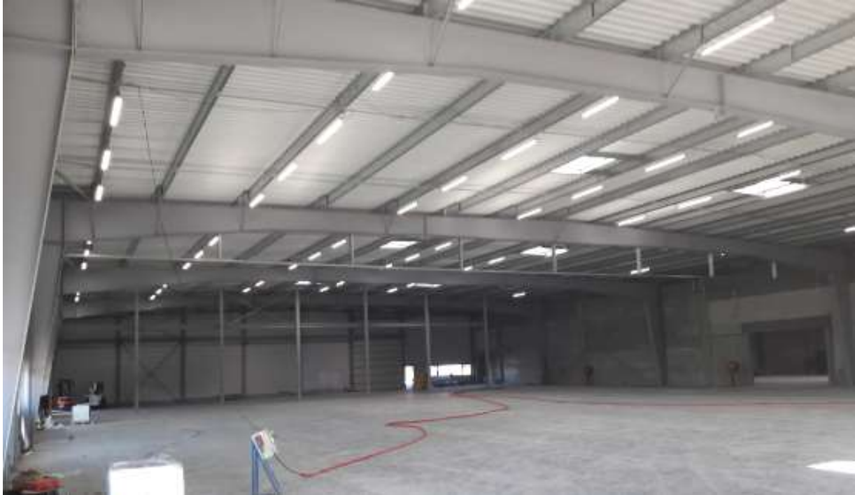
Figure 4: Portal frames with welded sections
