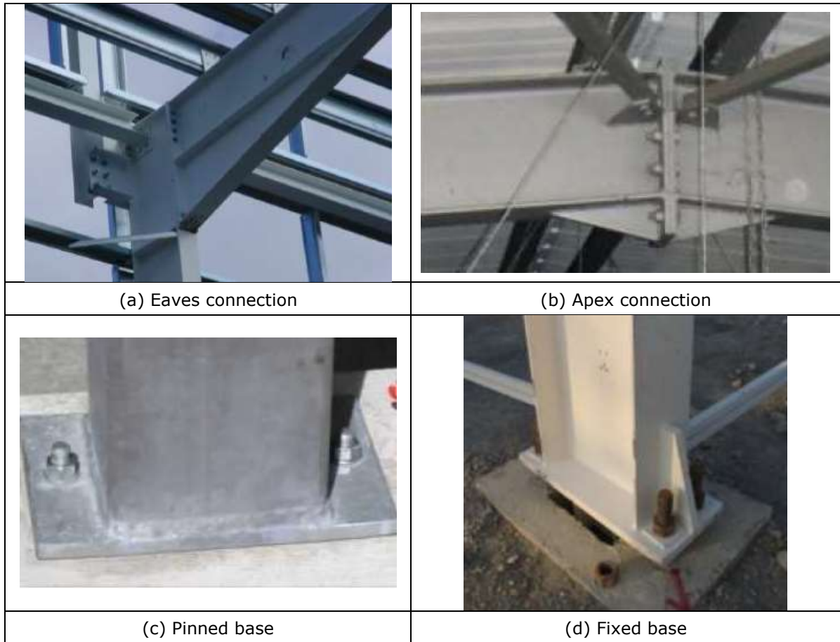
Figure 12: Typical connections in a portal frame (photos)
