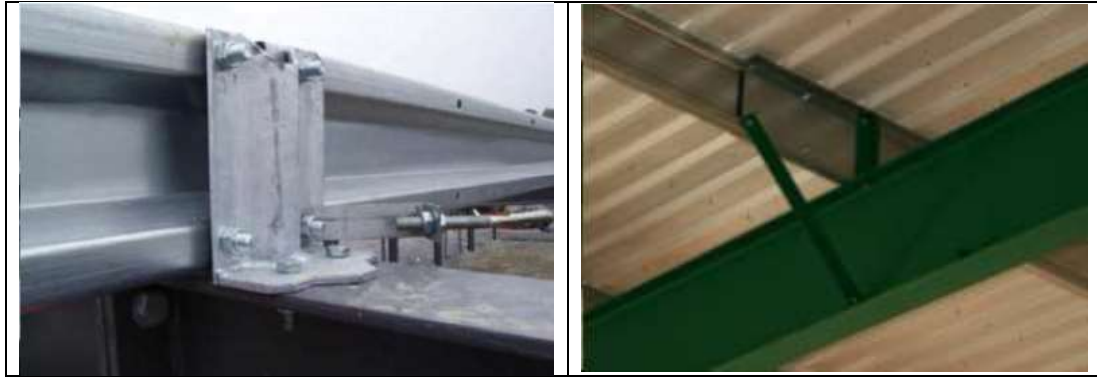
Figure 22: Typical connections for cold-form sections
