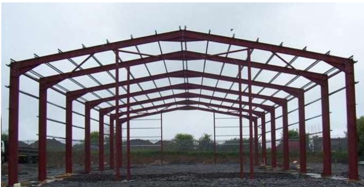
Figure 3: Portal frames with hot rolled sections
