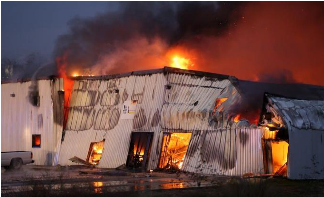
Figure 5.22: Steel façade collapsing with the building steel structure.
